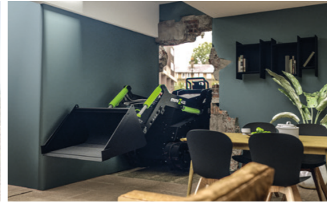
Interior construction / Demolition
