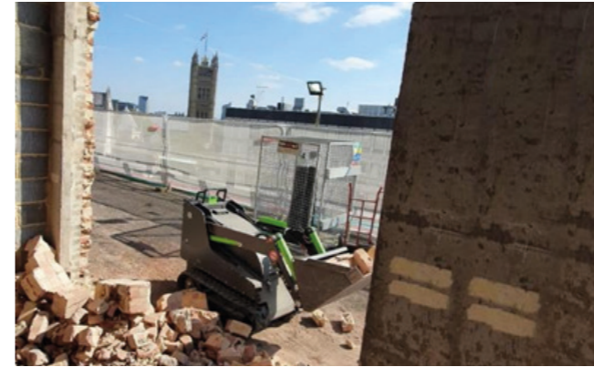
City construction / Demolition / Landscaping
